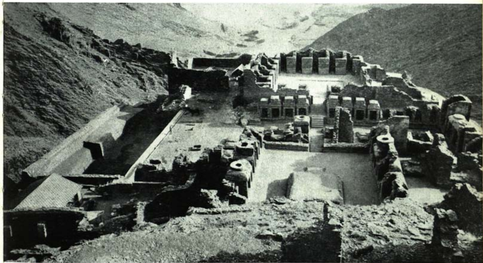
Fig. 2: Monastery of Takht-i-Behi near Peshawar, Pakistan
